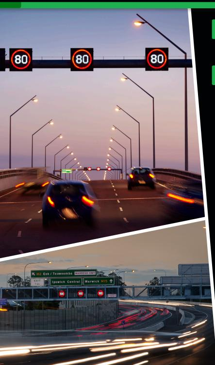
The LUMS combines the functionality of variable speed limit and lane control within one sign
